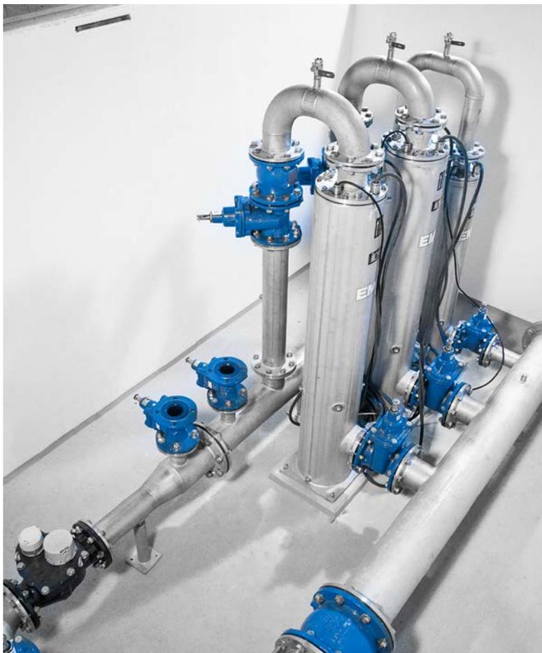
Drinking water: Branch and flushing shaft for two local networks UW 4266, installed condition
